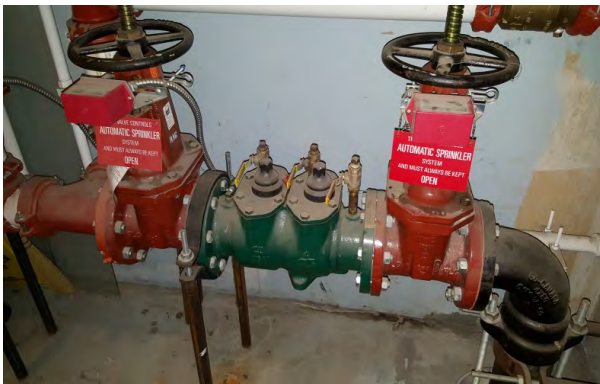
Main incoming fire service backflow preventer. Recommend yearly testing
