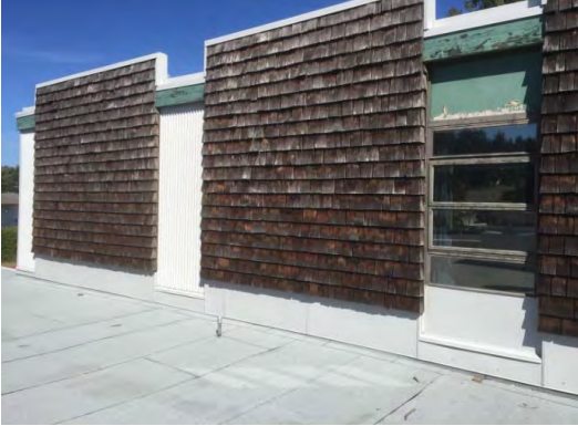
Photo B- Sections of roof where Block 2 and 3 abut have been re-flashed. No reports of problems with framing were identified in these locations.
