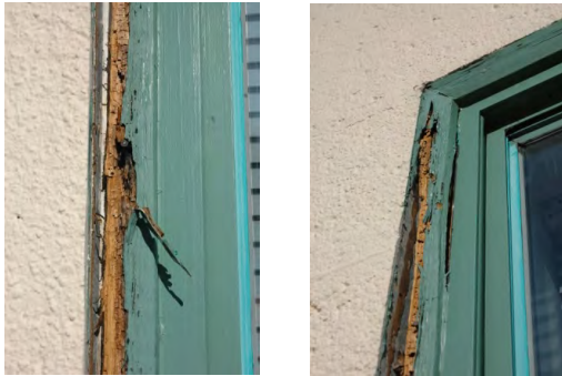
Deterioration of wood window trim on 1976 Block
