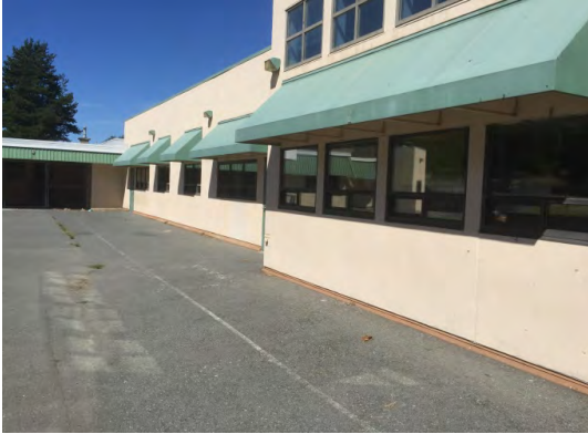
Photo A – Typical exterior view of southern exposure.
