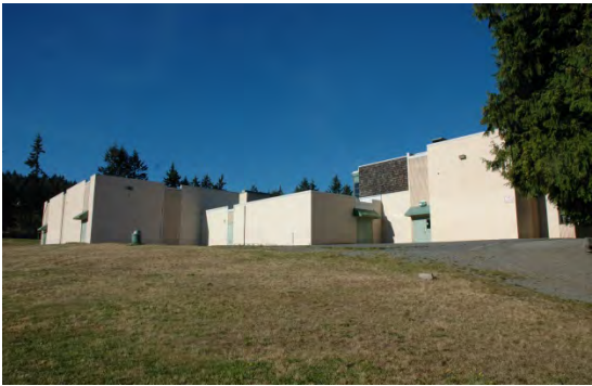
View of mostly concrete walls on south end of building.
