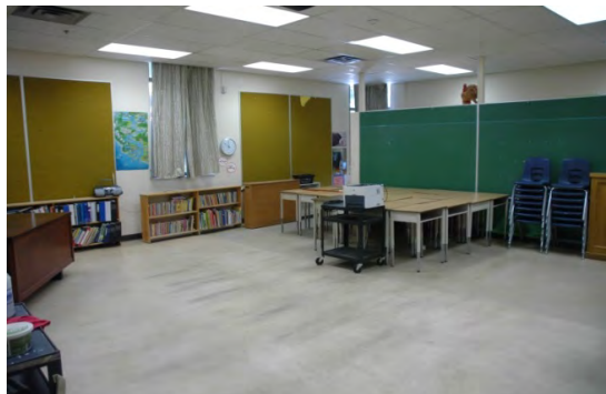
Millwork and fittings in the older blocks are generally of poor quality or condition.
