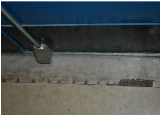
Patching at exterior door has chipped where floor is lifting. Nails used to prevent further buckling.
