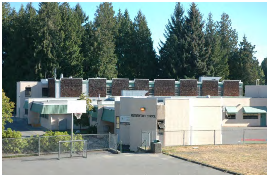
View of walls at north end of building.
