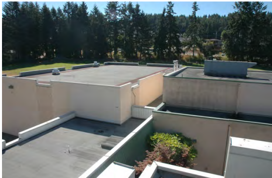
Roofscape at south end of building
