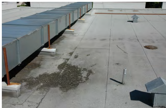
Some areas of the roof show signs of ponding. The 1981 roof is shown left.
