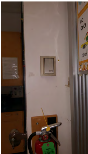
Thermostat for control of local heating system components
