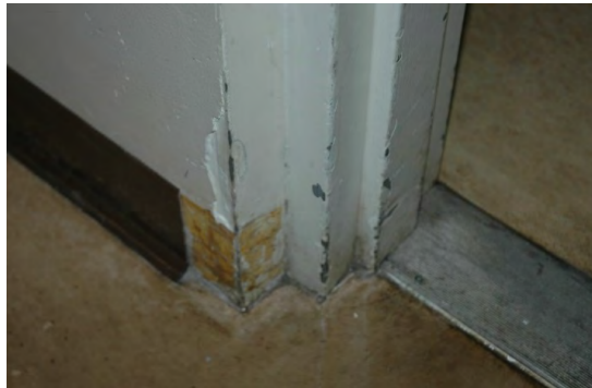
Damage to vinyl base, wall and door frame.
