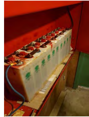
Figure 2: Fire Alarm Batteries
