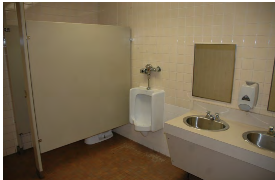
Washroom vanity faucet handles do not meet code for accessibility requirements. Metal toilet partitions used for non-accessible toilet stall. Urinal lacks code required grab bar and vanity mirror also doesn't meet code for accessibility.
