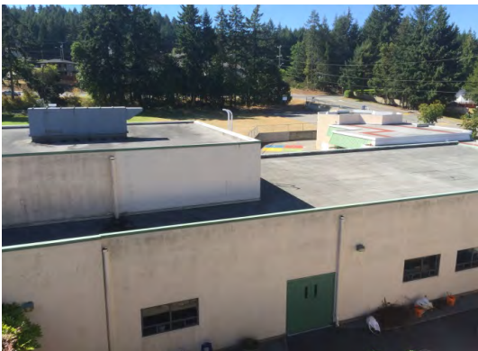
Photo C – Exterior view of north elevation of block. (Note staining and crazing of stucco)
