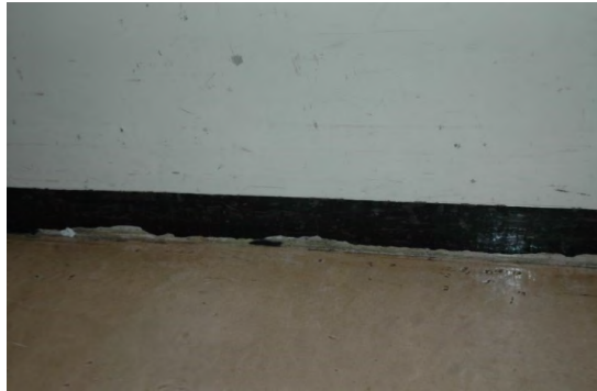
Chipped vinyl base in 1981 corridor.
