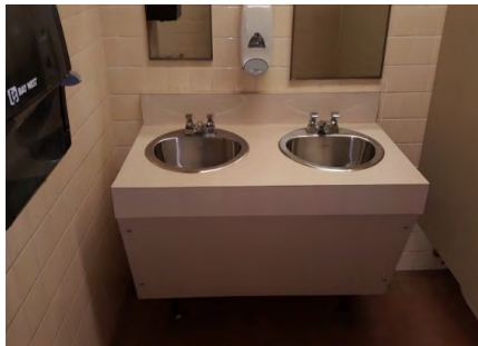
Washroom Lavatory (typical)
