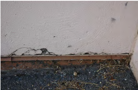
Stucco cracking and crumbling around wall base flashing in 1998 block
