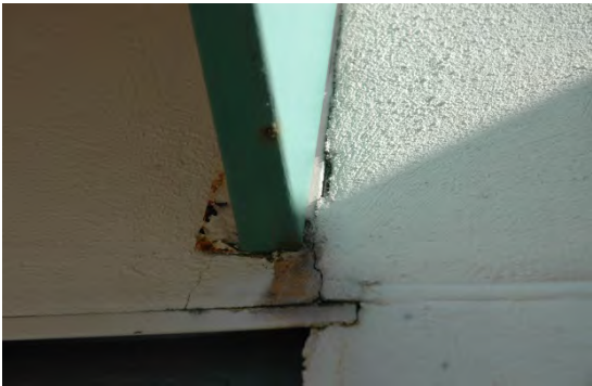
Stucco cracking and crumbling around canopy mounting bracket in 1998 block. Canopy support is rusting.
