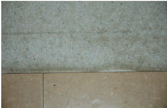
Junction of one old flooring to another with buckling at the joint.
