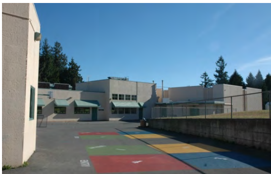
View of walls on west side of building.
