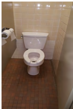
Washroom Water Closet (typical)
