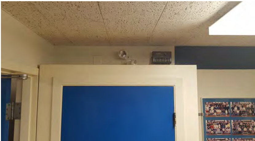
Figure 1: Improper Emergency Light Installation
