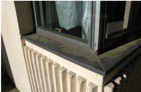
Typical window is single glazed with prefinished aluminum frame and sill flashings.
