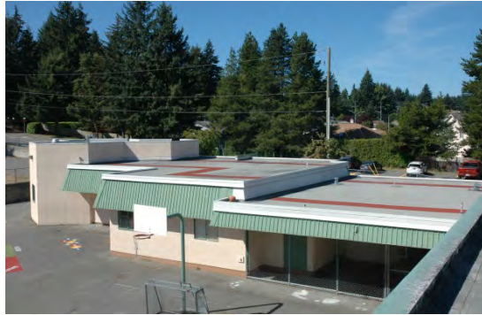
Roofscape at northwest corner of building
