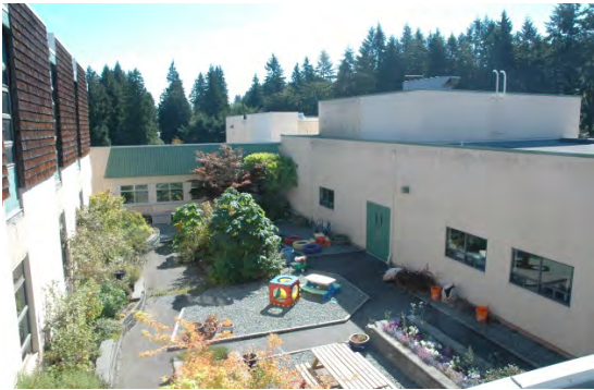
View of walls in courtyard.
