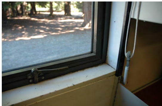
Evidence of condensation affecting wood window liner and sill.
