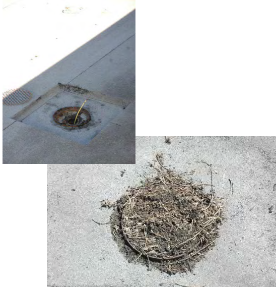
Several roof drains are missing strainers and strainers when present are flat and therefore prone to getting plugged with roof debris. Some roof drains are badly rusted, as shown in the photo far left.
