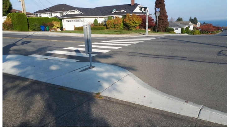
▲ New curb extensions and pedestrian beacons on Dover Rd.
