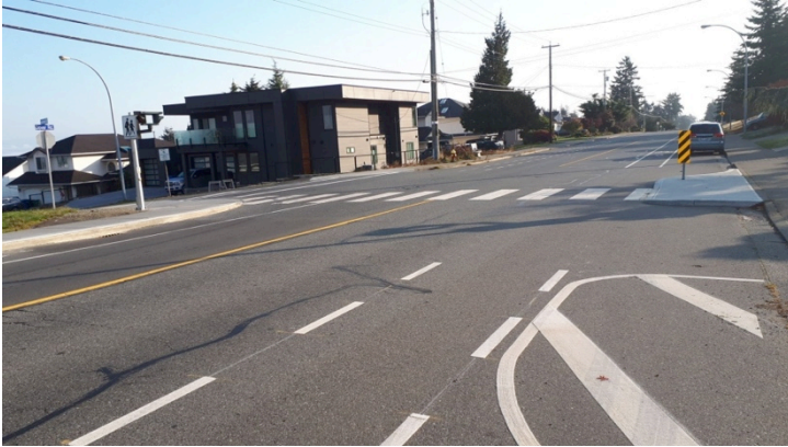
▲ New curb extensions and pedestrian beacons on Dover Rd.
