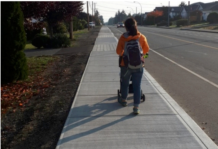
▲ New section of sidewalk on Dover Rd.
