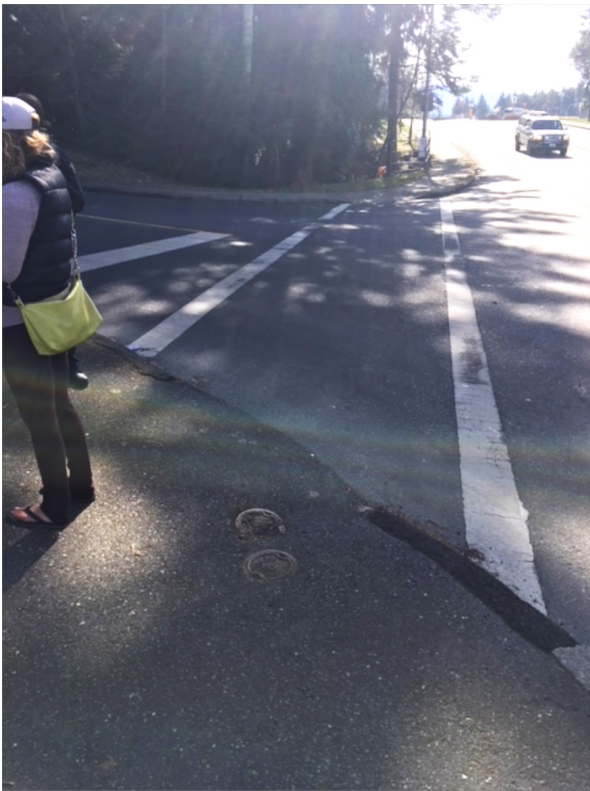
▲ Looking south across the crosswalk at the intersection of Nelson Rd. and Turner Rd.
