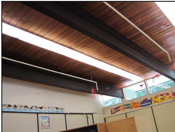
Fire Protection - Sprinkler Piping - No Seismic Restraint
