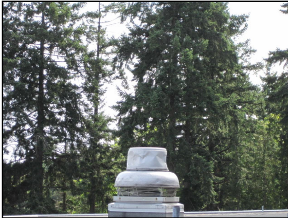
Exhaust System - General Building Renewal
