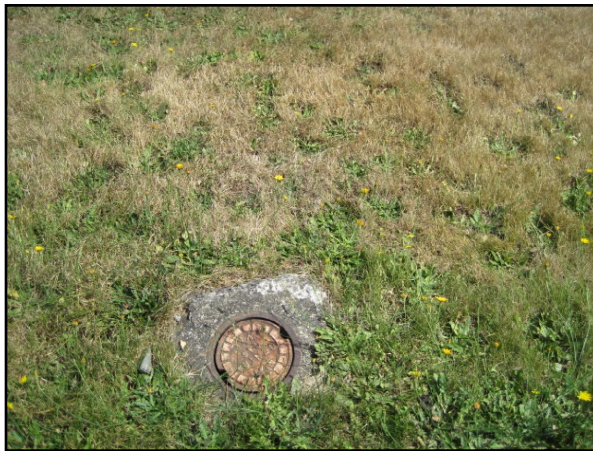
Underground Oil Tank - Steel Renewal
