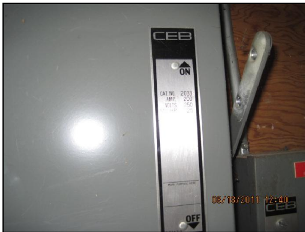
Main Electrical Service - 200A 120/240V Renewal
