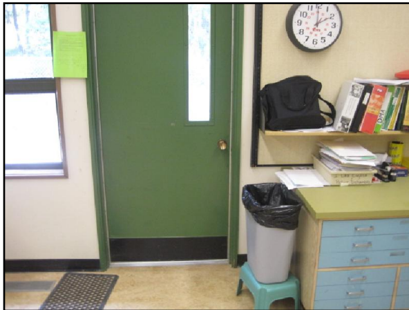
Interior Doors - Hardware Not Accessible
