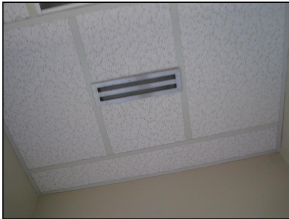
Distribution Systems - HVAC Ductwork Dirty
