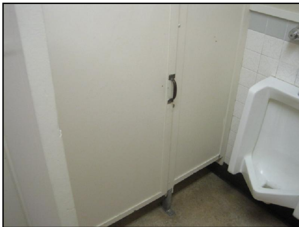
Wood Partitions Washrooms Renewal
