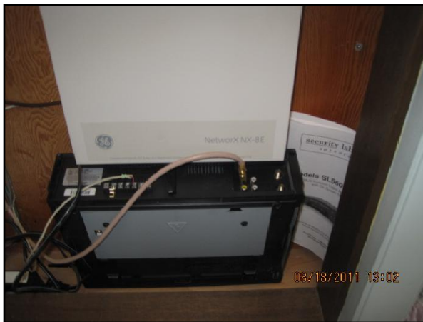
Security System Renewal
