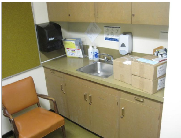
Casework - Elementary School Renewal Casework - Elementary School Renewal
