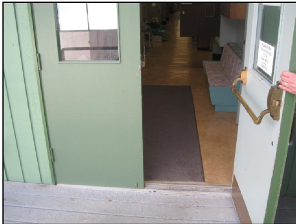
Exterior Doors - Automatic Door Openers Lacking at Entry
