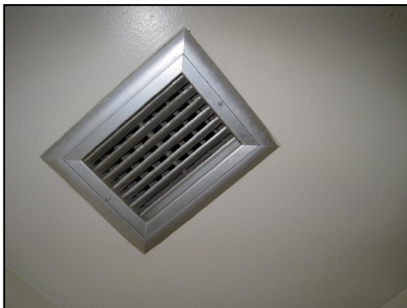
Distribution Systems - HVAC Ductwork Dirty
