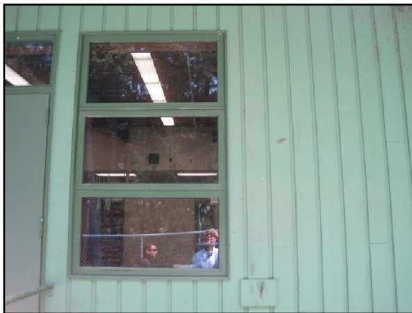
Windows - Metal Renewal
