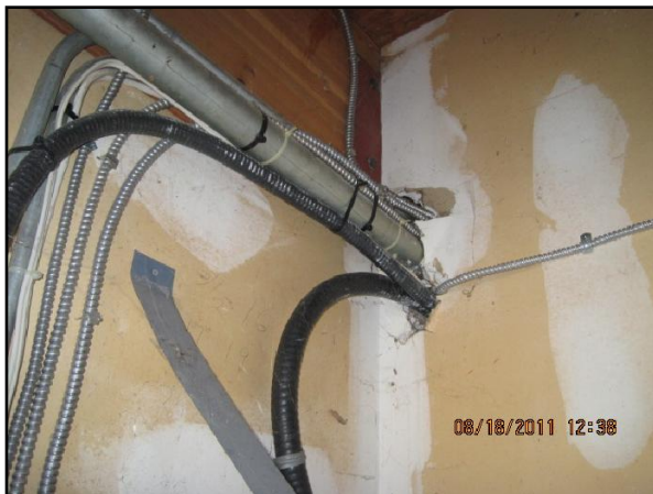
Electrical Conduits - Fire Stopping Not Installed
