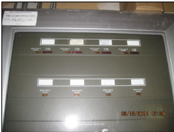
Fire Alarm System Renewal
