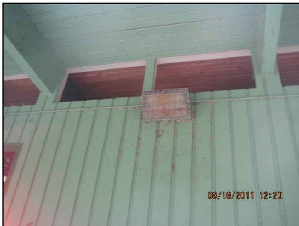
Lighting - Exterior Renewal
