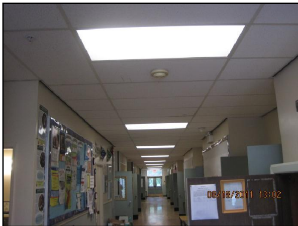
Non-Seismic Luminaire - Corridors
