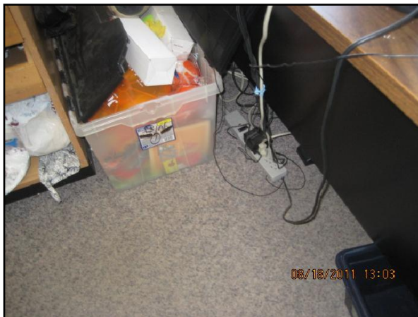
Branch Wiring Devices - Insufficient Quantity of Receptacles
