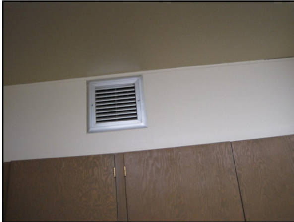
Distribution Systems - HVAC Ductwork Dirty
