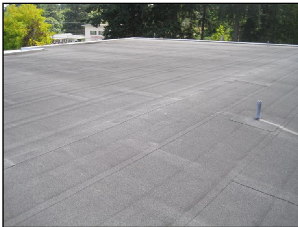
SBS Modified Bitumen Membrane Renewal
