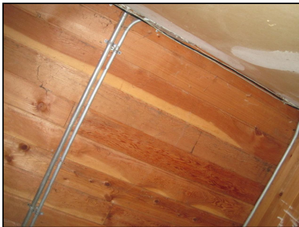
Distribution Systems - Ventilation System Not Installed
