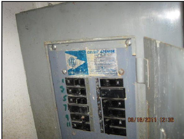
Panelboards, Feeders and Disconnects - 120/240V Renewal
