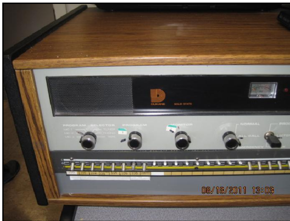
Public Address System Renewal
