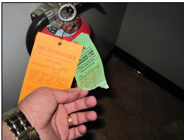
Various Mechanical Deficiencies
