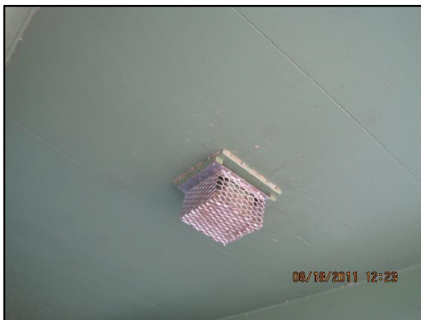
Lighting - Exterior Renewal
